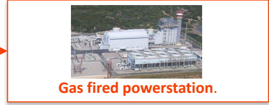
CHP combined heat and power,
