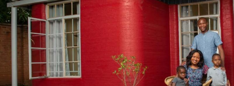
We printed a 36m<sup>2</sup> house in less than 12 hours Starting price is at 9,500 USD A 3D printed house emits 70% less CO2 than a conventional, burnt brick house in Malawi
