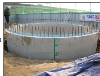
Install the caisson
