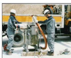
Impervious material injection
