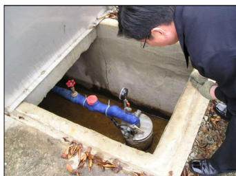
Inspection of pipe
