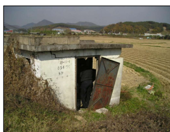
Check of well house
