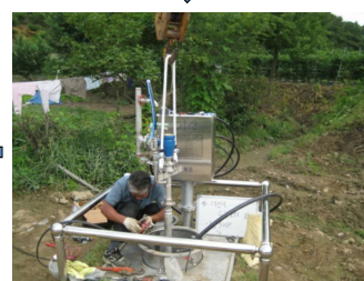
Installing well protection guide
