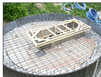
Completion of installation
