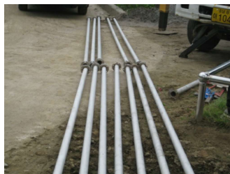
Installing of pipe
