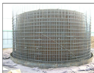
Install the rebar and reinforced concrete
