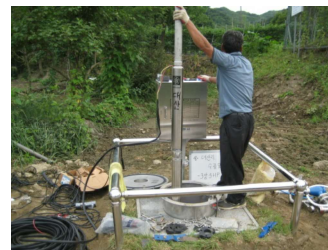
Installing submersible pump
