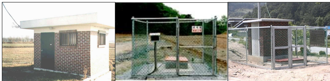
Groundwater pollution prevention facility
