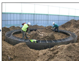
Install the sue steel sheet
