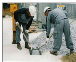
Insert backfill material into well
