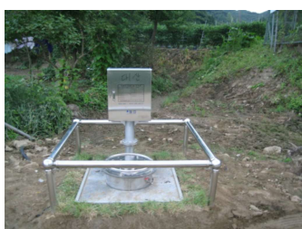
Completed well facility
